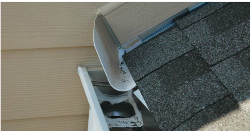
With horizontal siding, the author installs a trim board along the rake, keeping it a minimum of 1 inch above the roofing.
