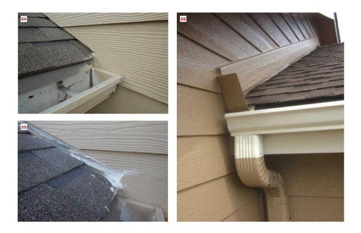
and it also created an inferior caulk fillet that failed quickly and allowed water to seep into the joint when the siding boards contracted.
