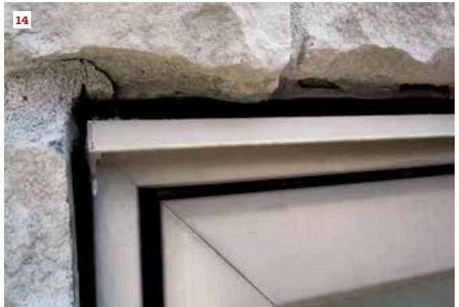
We have to constantly remind ourselves that ACMV absorbs and holds a lot of water, so we need to do everything possible to avoid loading the stone with water. Wide overhangs and meticulous detailing on gutters and valleys are critically important.
