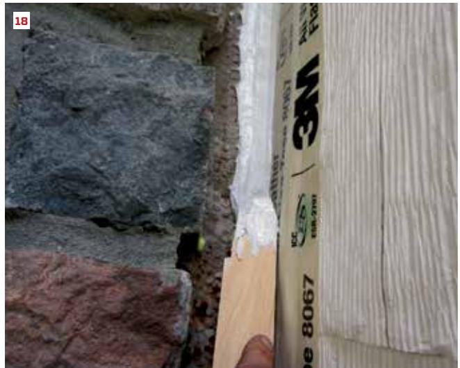
thermal expansion of dissimilar materials. What usually happens is that the masons will simply fill the gap between the window and the stone with mortar, and the mortar cracks almost immediately. If nothing else, this looks bad. But usually the wall is not drainable, so the crack also allows for the speedy flow of water into the wall.
