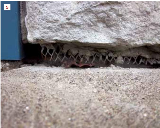
to drain to the outside from behind the brick. To create a drainable system, I always use a rainscreen material, such as Keene Dri-wall (keenebuilding.com), which is shown in the photos for this job. Recently I have been using MTI Cavity Gravity (mtidry.com), which was developed for brick walls but also works with EIFS and ACMV. It stays rigid, which makes applying the lath easier and helps to maintain an even thickness for the scratch coat.
